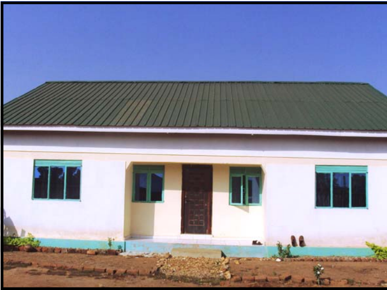
The facade of the new MRDA Guest House
