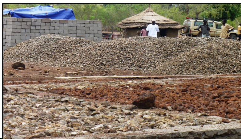
Construction going on at Lunjini Primary School, Kediba Payam, Mundri East
